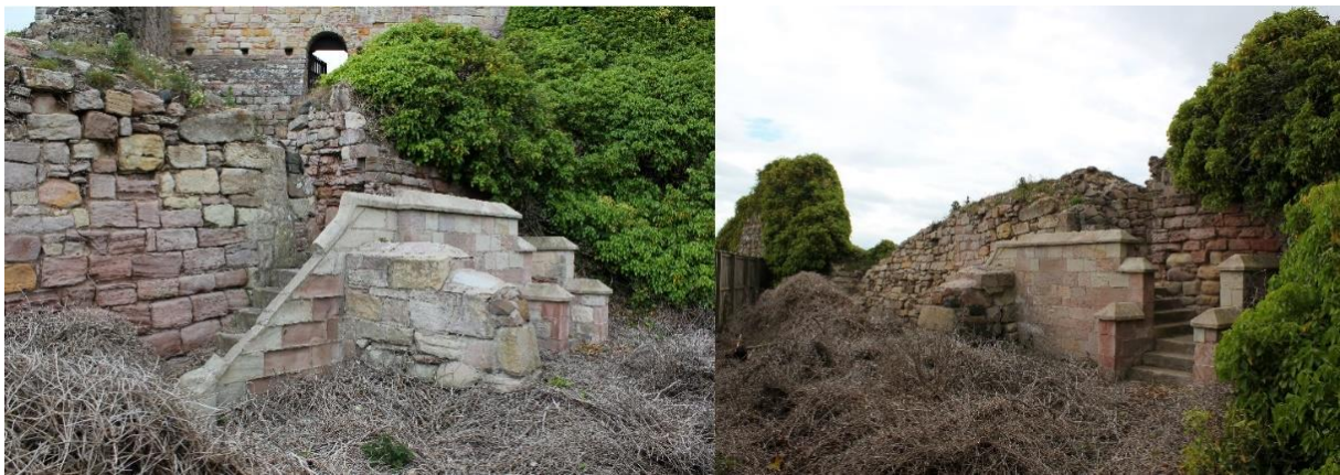
Figure 4: Two views of the late post medieval steps that approach the postern gate, facing north-east on right and north-west on left.
