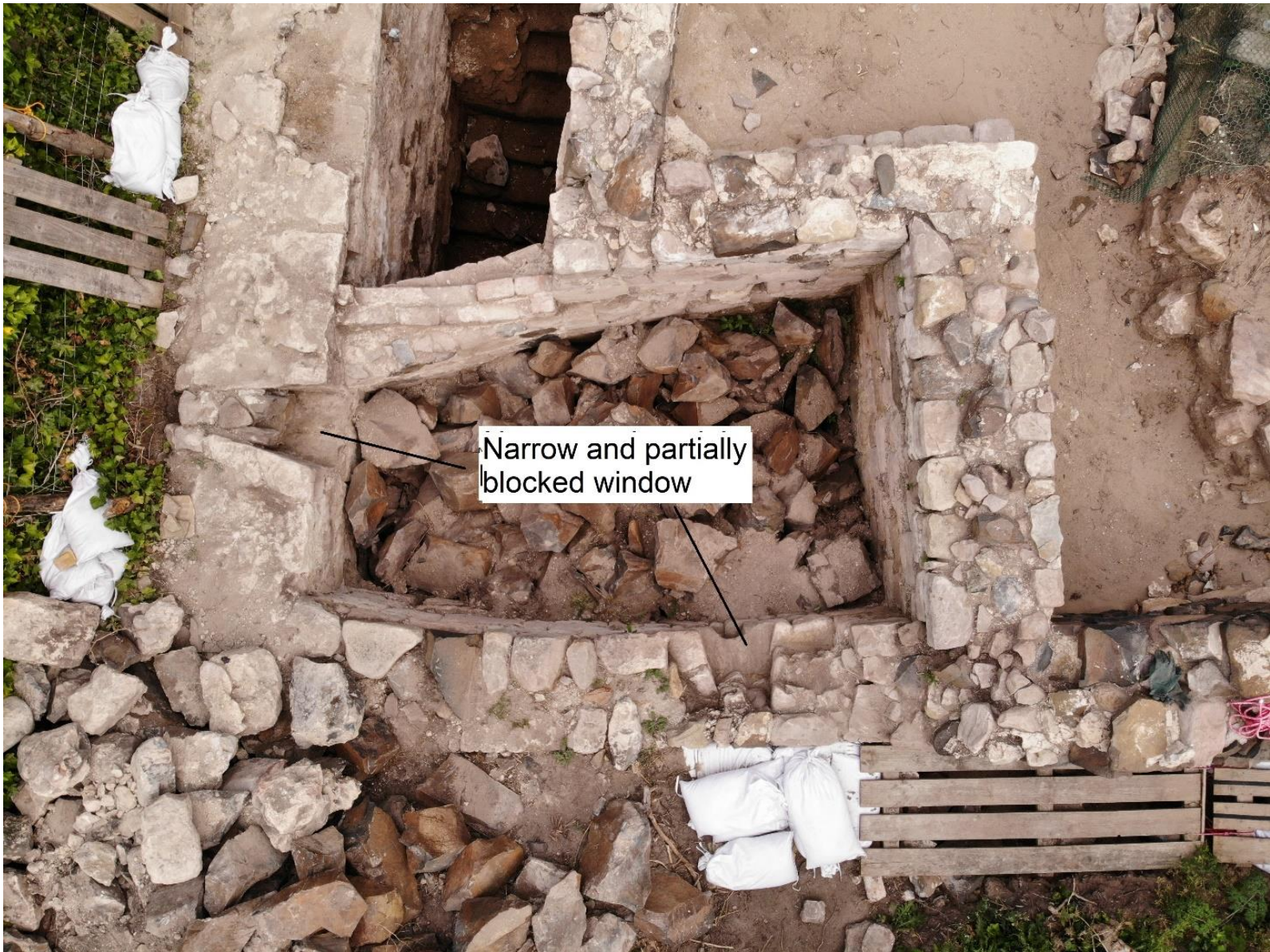
Figure 10: The tower from above showing the partially blocked narrow windows, facing east
