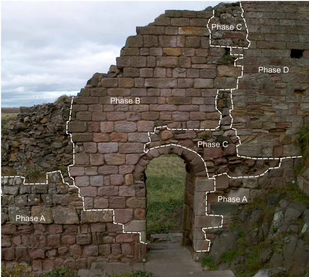
Figure 5: The narrow 'Wing Wall' showing the narrow archway and multiple phases of construction, facing north-west
