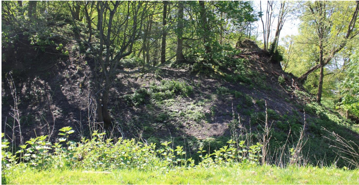
Figure 4. The entrance to the inner bailey viewed from the north-east, from a position in the outer bailey.
