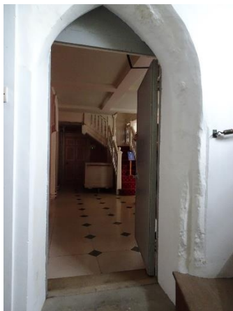
Fig. 102: Doorway F17-5 between the Great Hall and spiral stair SSB, looking south into the Hall
