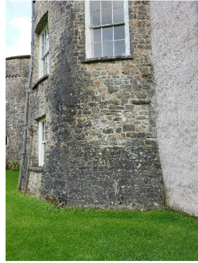
Fig. 81: Northwest face of the Northwest Tower, showing blocked window G11a-4
