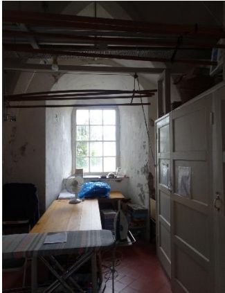
Fig. 76: Southern undercroft central bay G10b, looking south
