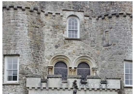
Fig. 161: Gatehouse frontage, looking west showing infilled outer arch, and blocked loops T31-1 and T31-2 either side
