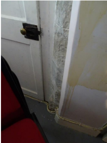
Fig. 106: Doorway F18a-3 showing pyramidal chamfer-stop, looking west
