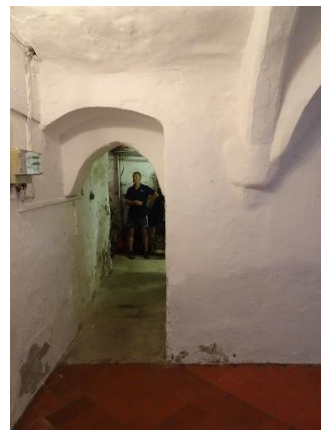
Fig. 69: Entry G10a-1, between north and south undercrofts, looking south
