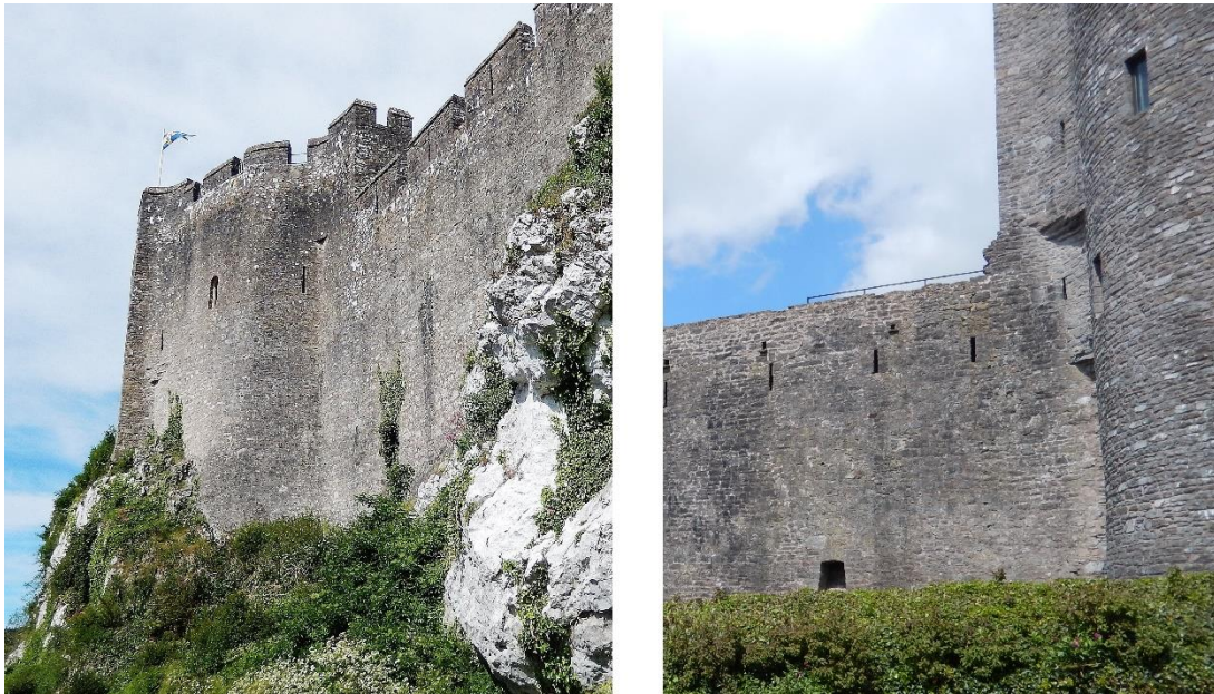
Fig. 203: Sinuous angles and squinching in work from the 1250s at Pembroke Castle
