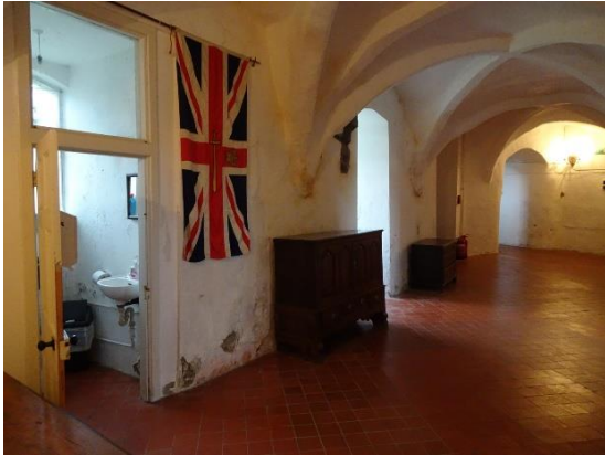
Fig. 66: Northern undercroft G9, looking northeast; entry G9-1 at far end
