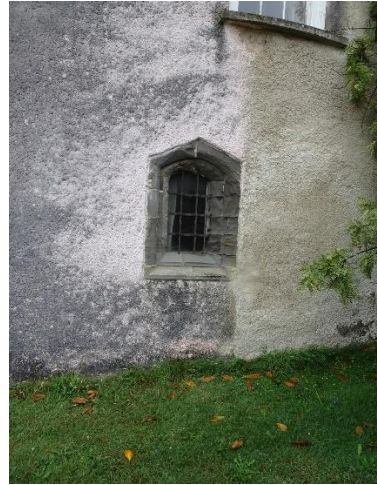
Fig. 55: Southeast Tower light G7b-2 from the exterior, showing modern surround
