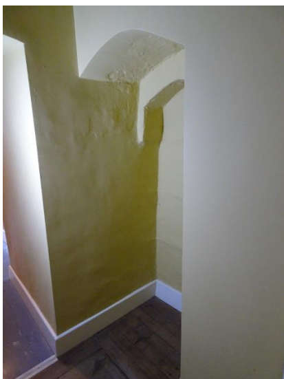
Fig. 90: Former northern doorway to the portcullis chamber F12b-1, looking southeast
