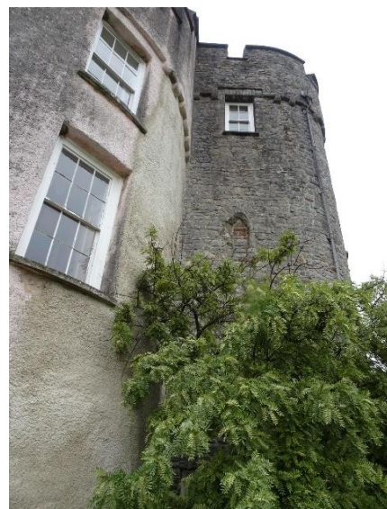
Fig. 122: External view of south gate-tower, showing blocked second-floor light S24-3 with medieval surround
