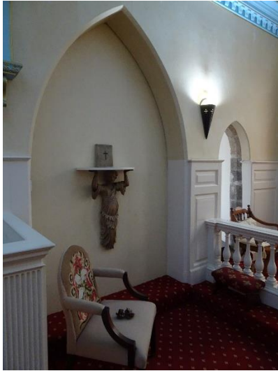
Fig. 127: Early nineteenth-century organ recess S23-3, looking northeast
