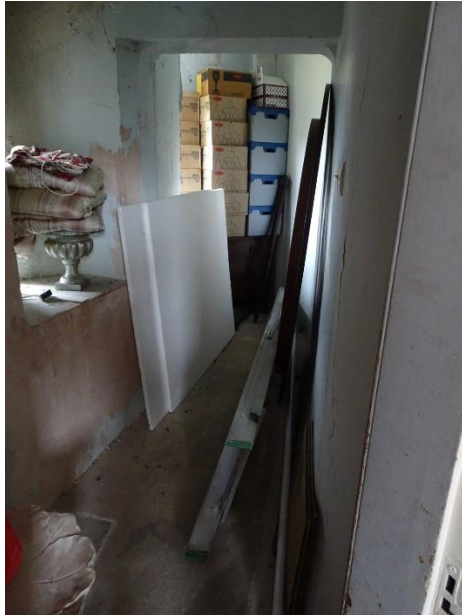
Fig. 111: Interior of southwest passage F20, looking southwest
