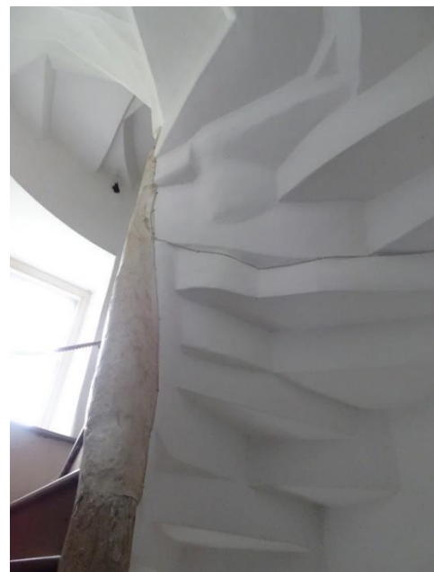
Fig. 63: Spiral stair SSB, looking up at the 'crow's foot' risers
