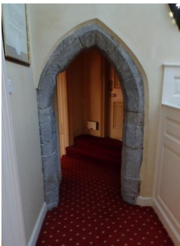
Fig. 129: Medieval doorway S23-4, between chapel S23 and Northeast Tower, looking north
