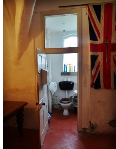
Fig. 73: North wall west opening G9-4, looking north
