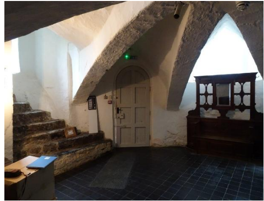
Fig. 49: Northeast Tower room G6, looking southwest, showing post-medieval entry G6-5 onto spiral stair SSB
