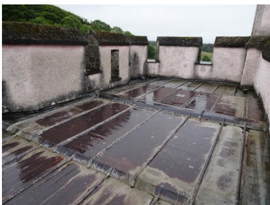
Fig. 172: Gatehouse roof looking southeast, showing open parapet loop
