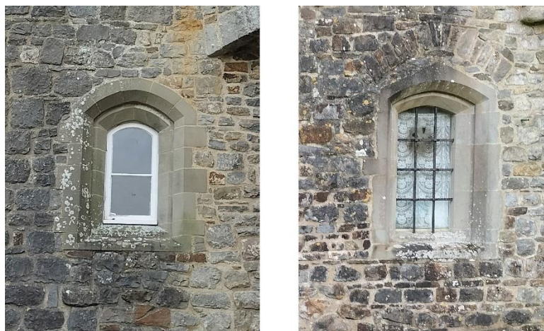
Fig. 231: 1960s double-chamfered surrounds: windows F13-2 and G9-4
