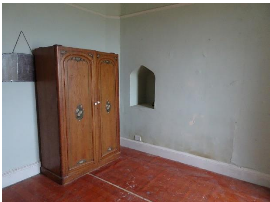
Fig. 162: Gatehouse southern third-floor room showing east wall recess T31-3, looking northeast
