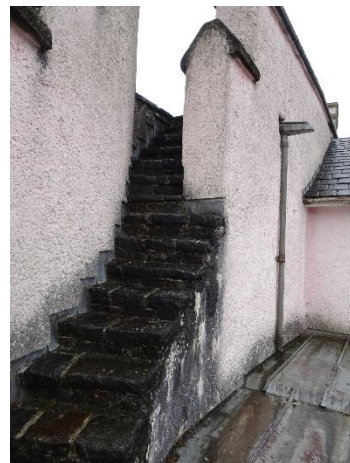
Fig. 163: Steps up from Northeast Tower parapet to gatehouse parapet, looking southeast
