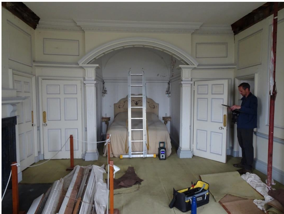
Fig. 215: Southeast Tower second-floor bedroom S30d, looking north showing early eighteenth century fittings including 'vaulted' bed recess
