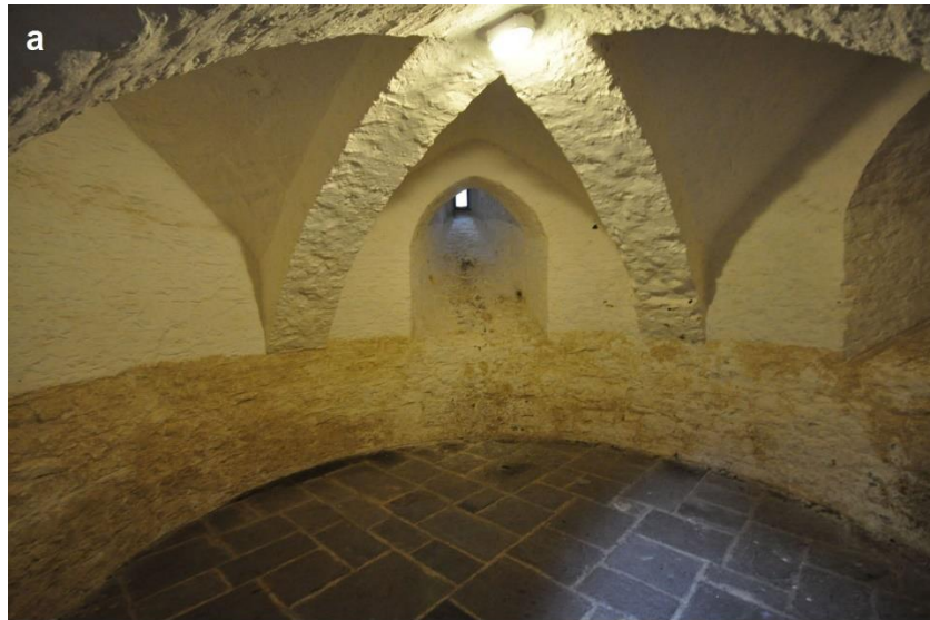
Fig. 196: Low rib-vaults with a deep extrados at a) Castell Coch (Glam.), late 1260s-70s; b) Picton Castle northeast tower
