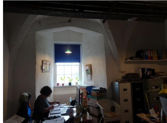
Fig. 77: Southern undercroft western bay G10c, looking south
