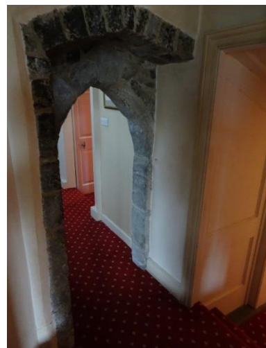
Fig. 130: Medieval doorway S23-4, between chapel S23 and Northeast Tower, looking southwest
