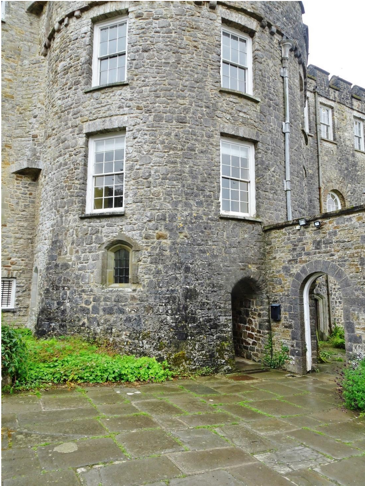
Fig. 22: Photo of Picton Castle Northeast Tower from the northeast (June 2023)
