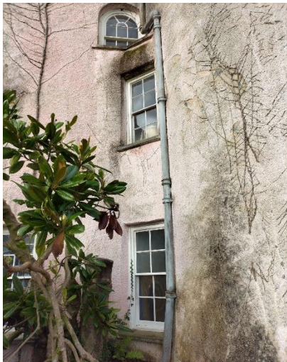
Fig. 58: Southeast Tower exterior showing windows G7a-1, F18a-1 and S28-2, looking northeast
