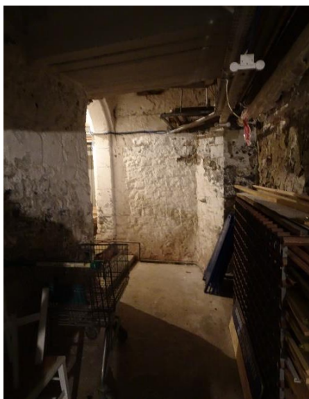
Fig. 52: Southeast Tower room G7a, looking northeast, showing gate-passage doorway G2b-4
