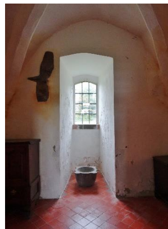
Fig. 71: North wall opening G9-3, looking north showing remains of ?surround
