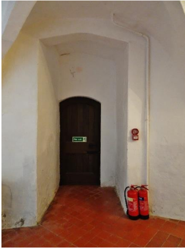
Fig. 72: North wall east opening G9-2, looking north
