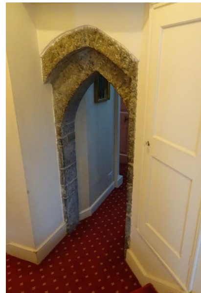
Fig. 134: Medieval doorway S23-5, between chapel S23 and Southeast Tower, looking northwest
