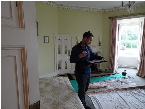
Fig. 142: Southeast Tower room S27, looking east towards entry S27-1
