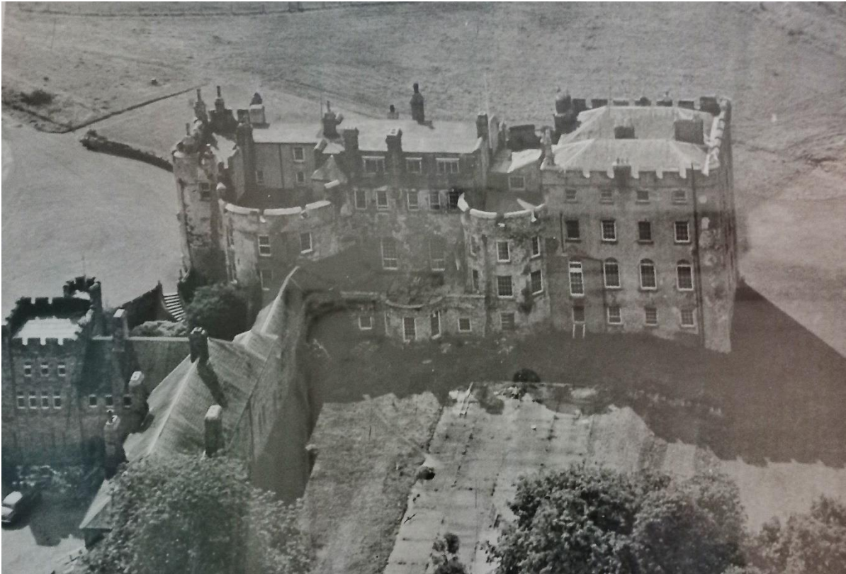
Fig. 213: Aerial photo of Picton Castle, looking south, taken during the 1950s (Picton Castle Trust)
