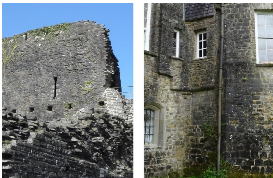
Fig. 194: Fishtail loops at a) Caerphilly Castle (Glam.), 1270s (photo Neil Guy); b) Picton Castle, Northwest Tower east face (beneath sill of centre window F19-2)
