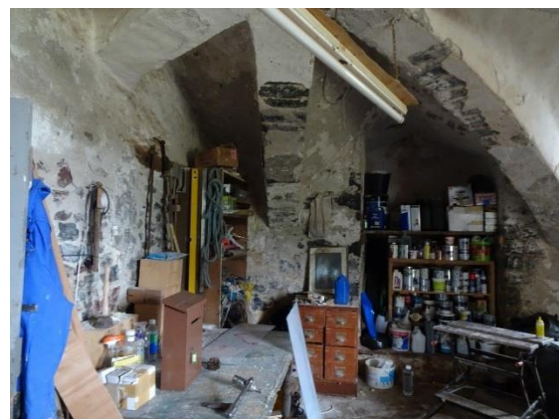
Fig. 53: Southeast Tower room G7b, looking east, showing blocked light G7b-1
