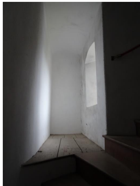
Fig. 150: Mural chamber S29, looking west from spiral stair SSB
