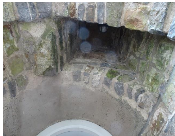
Fig. 51: Head of Northeast Tower doorway G6-3, showing blocked shaft
