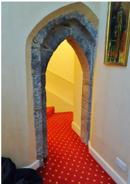
Fig. 133: Medieval doorway S23-5, between chapel S23 and Southeast Tower, looking southwest
