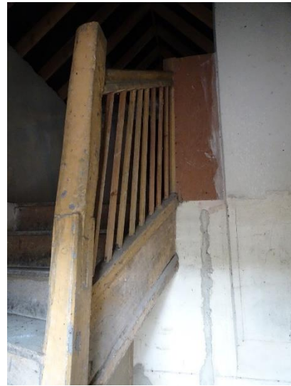
Fig. 167: Continuation of spiral stair SSB towards attic, looking southeast
