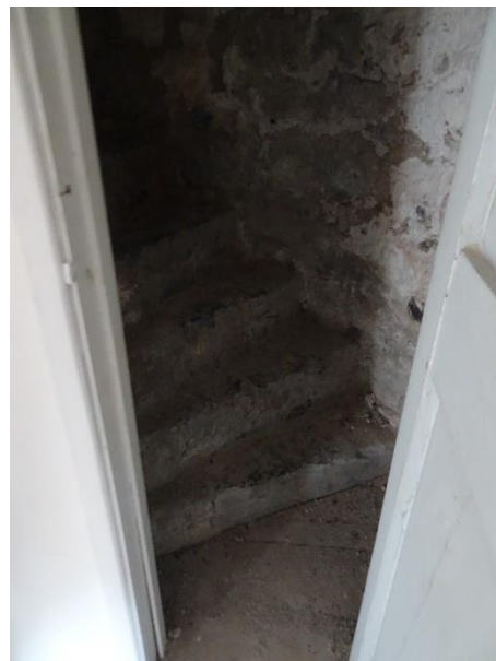
Fig. 152: Southwest Tower room S30d: spiral stair SSC, looking north
