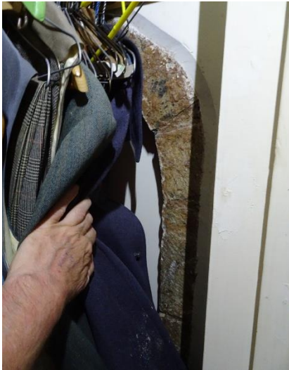
Fig. 139: The head of blocked medieval passage doorway S26-2, now in a cupboard in room S25, looking northwest
