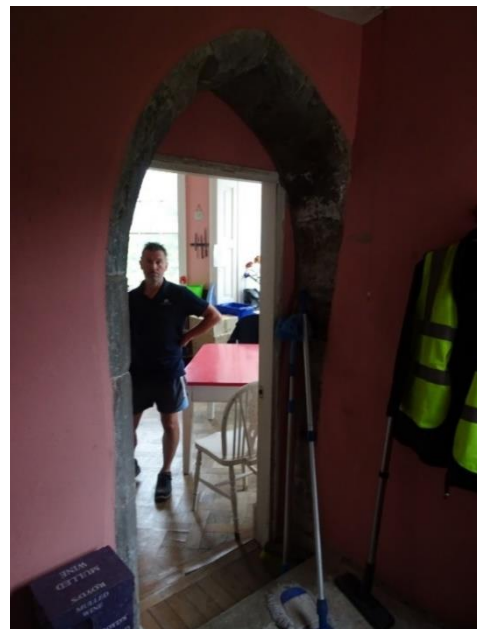
Fig. 109: Northwest passage F19 – doorway F19-3 into the Northwest Tower, looking northwest
