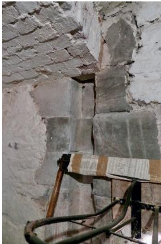
Fig. 33: Portcullis groove G2a-2 in passage south wall
