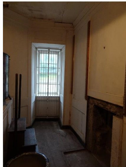
Fig. 93: South gatehouse tower, looking east showing south wall fireplace F14-2
