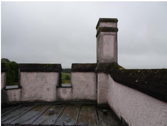
Fig. 160: Summit of gatehouse, looking southwest showing roof, parapet and chimney T31-9
