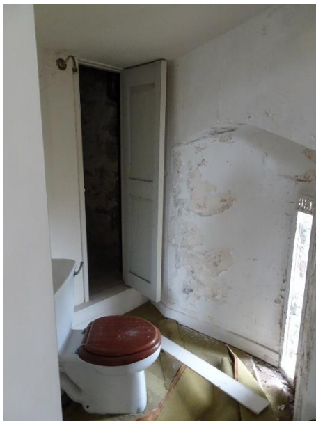
Fig. 151: Southwest Tower room S30d: passage to spiral stair SSC, looking northeast
