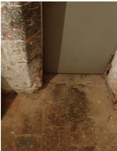
Fig. 38: Pyramidal chamfer-stop in passage doorway G2b-1, looking north
