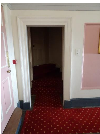
Fig. 146: Doorway S25-6 from Great Hall gallery to Northeast Tower, looking east
