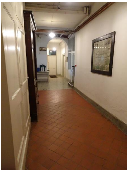
Fig. 78: Corridor G11d between the Western Towers, looking west into the 1790s Western Block
