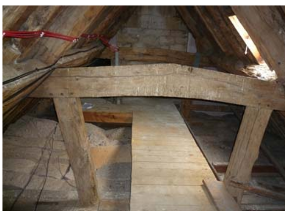
Photo 20: East range – truss 4 with no diminished principal rafters
