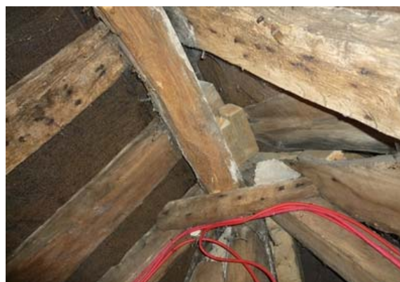
Photo 6: West range – ridge purlin
