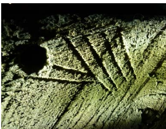
Photo 23: East range – a re-used timber showing 45° trestle saw marks and scribed carpenter's marks
