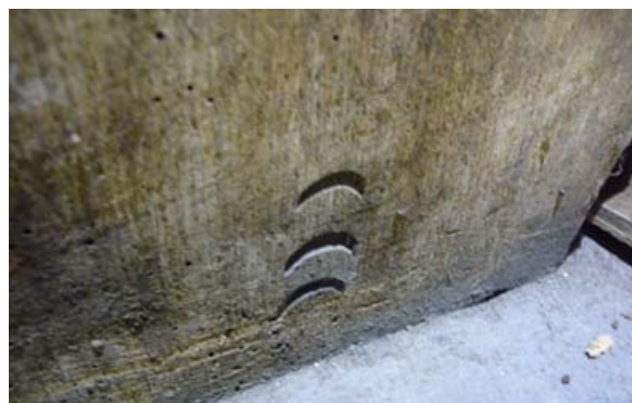
Photo 16: North range – curved chiselled carpenter's marks
