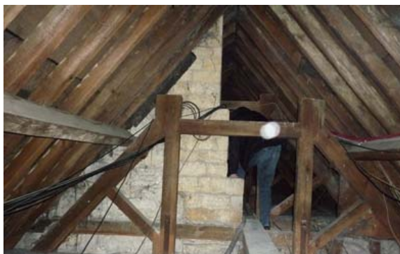
Photo 17: North range – later pine trusses
