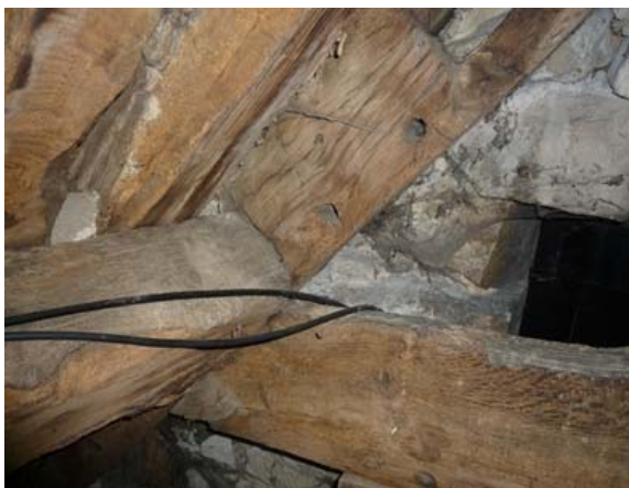
Photo 21: East range – truss 1 showing re-used principal rafter with empty mortises
