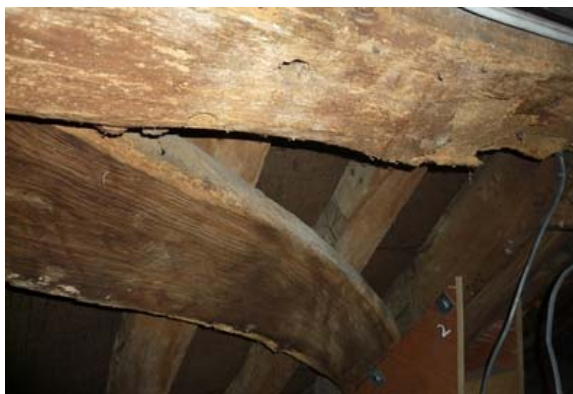
Photo 7: West range – a re-used curved windbrace
