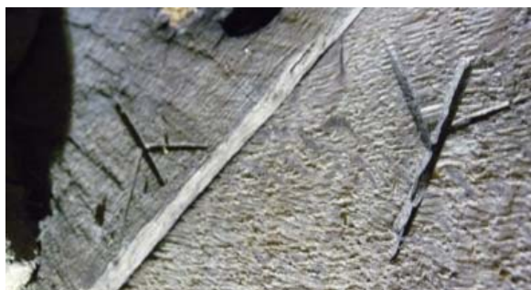
Photo 12: West range – chiselled carpenter's mark on truss
