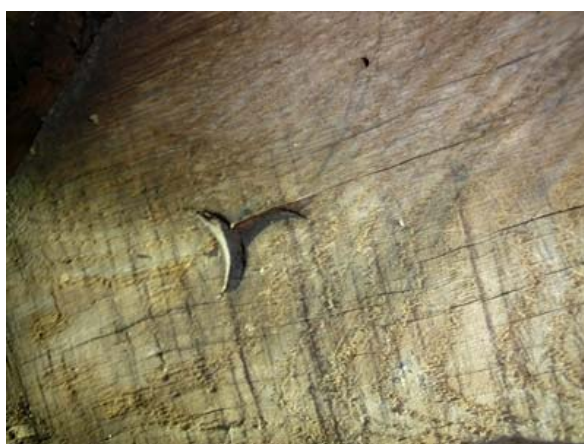
Photo 24: East range – a non-re-used timber showing 90° pit saw marks and a curved chiselled carpenter's mark
