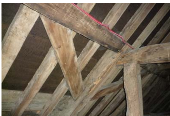
Photo 13: North range – queen-strut roof with clasped purlins supported by straight windbraces
