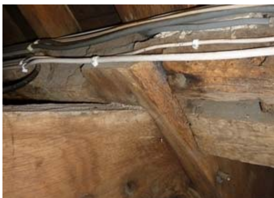
Photo 5: West range – diminished principal rafter
