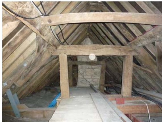
Photo 4: West range – raking queen-strut roof with clasped purlins
