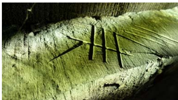
Photo 11: West range – complex chiselled carpenter's mark on rafter
