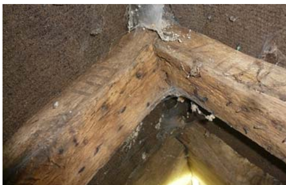
Photo 15: North range – chiselled carpenter's marks
