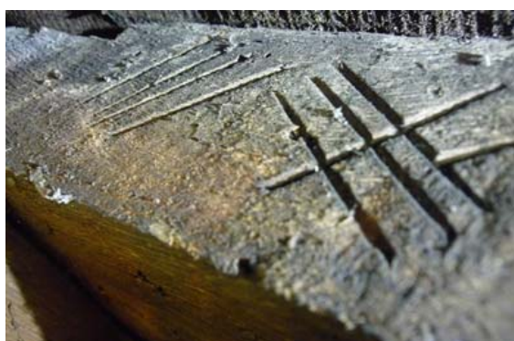
Photo 10: West range – complex chiselled carpenter's mark on rafter
