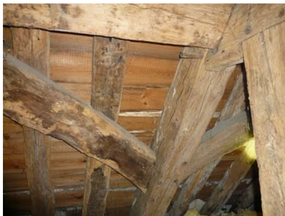
Photo 22: East range – smoke-blackened re-used curved windbrace (left)
